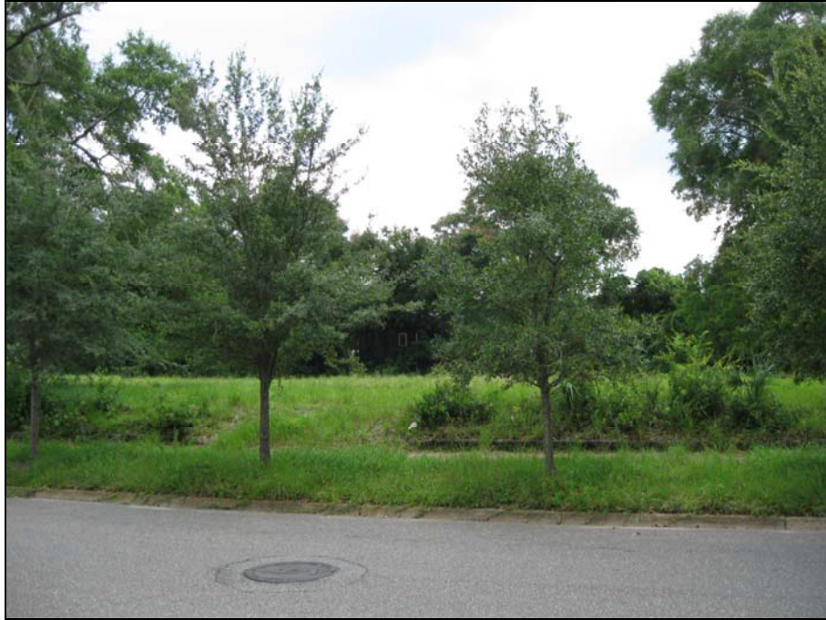
Elevation change between the sidewalk and grade.
